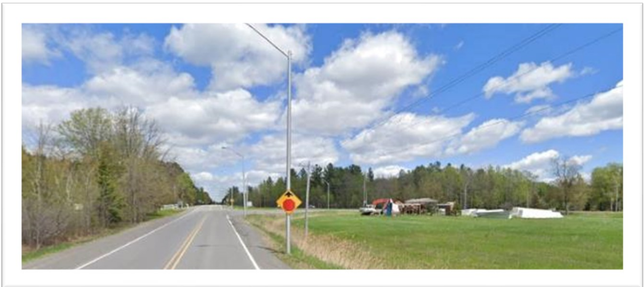
Figure 16: Intersection at Beckett’s Landing – no arrow pointing to Kemptville
